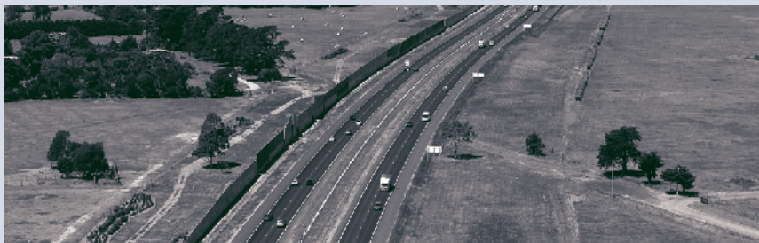
Pakenham Bypass looking east and showing noise walls (Photo DITRD/LG)
