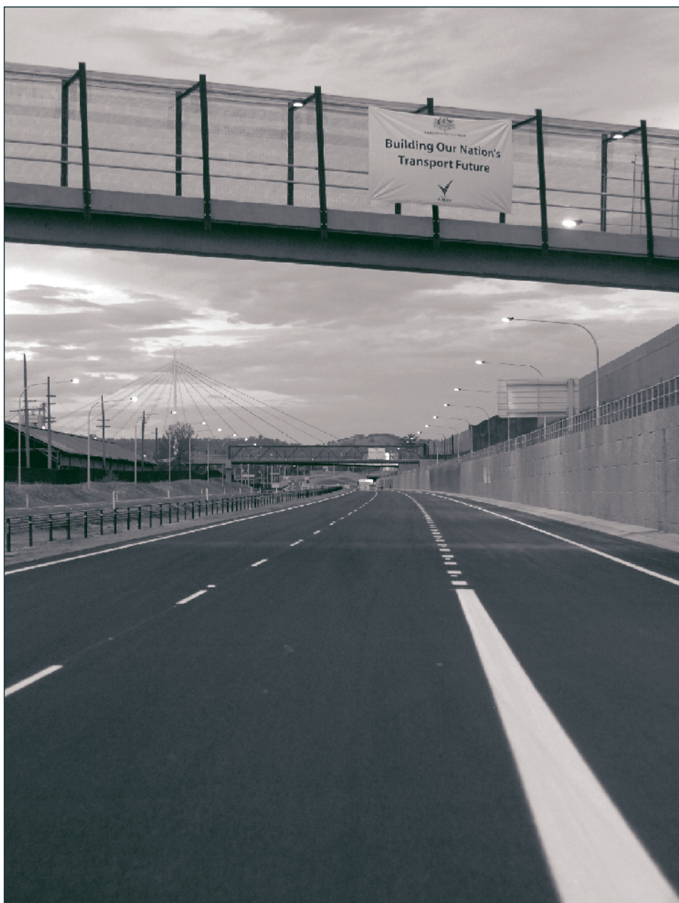
Albury-Wodonga upgrade: Improving vehicle efficiency and pedestrian safety (Photo DITRDG)
