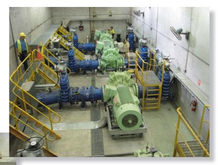
One of the unique features of this project is that due to the pump station's position it can actually supply reasonable quantities of water (300L/S) without the pumps actually running. The pump sets were progressively replaced and work can be seen still going on in the photos.
