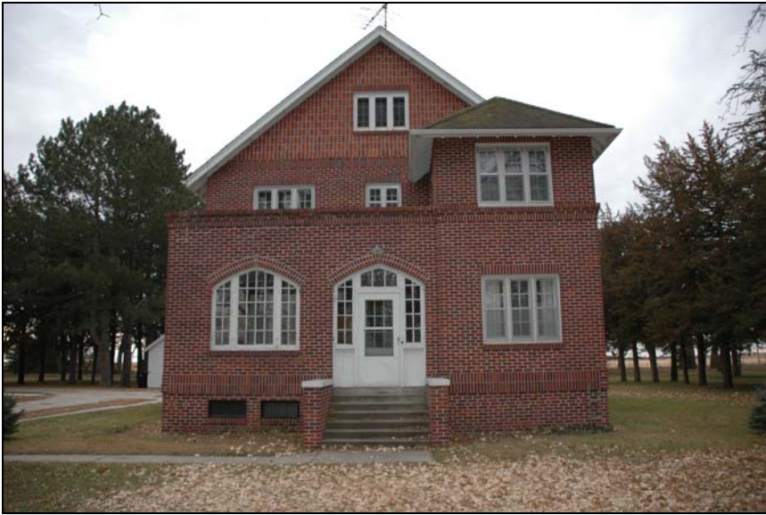
St. Anselm's Church, Rectory & Parish Hall Photo by Stacy Stupka-Burda Photo 7 of 12 – View of rectory, front façade, looking S
