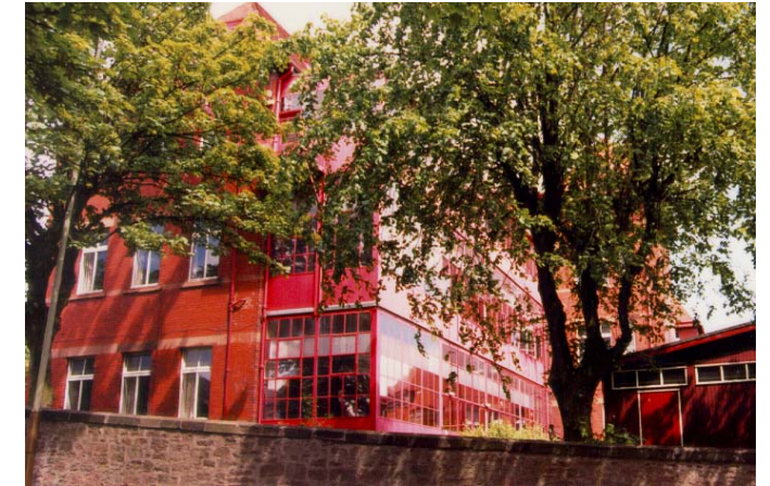
2 Caird Wing Balconies
