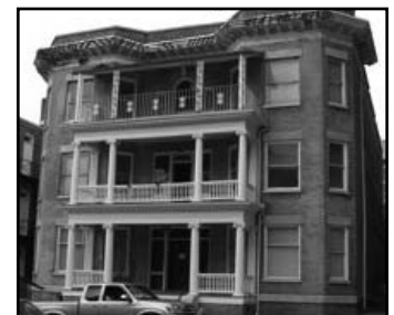
The Glencoe Building
