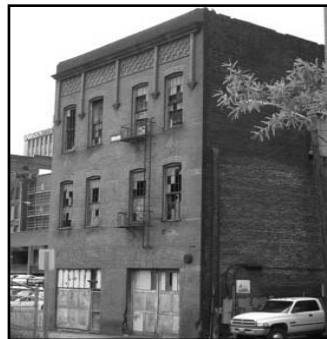
Cal Johnson Building
