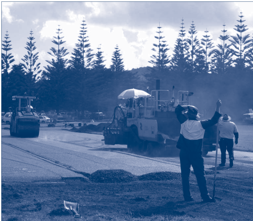
Airport runway upgrade works (Photo courtesy Norfolk Island Government)
