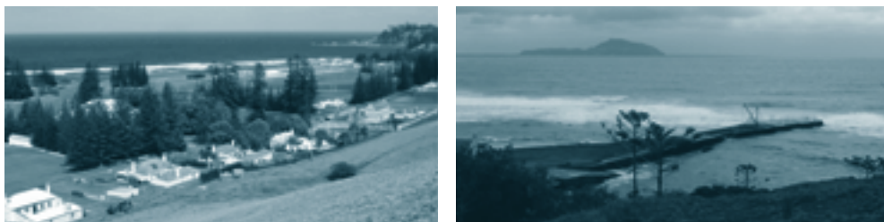
Above: Norfolk Island contains the best remaining examples of Georgian architecture in Australia but provides a challenging environment for conservators (Photos Jim Mallett DOTARS)
