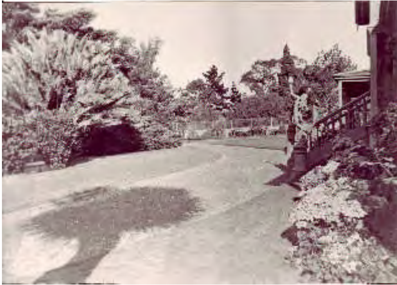
Figure 19 View of The Cliffe Grounds, 1920s Courtesy of PLC archives
