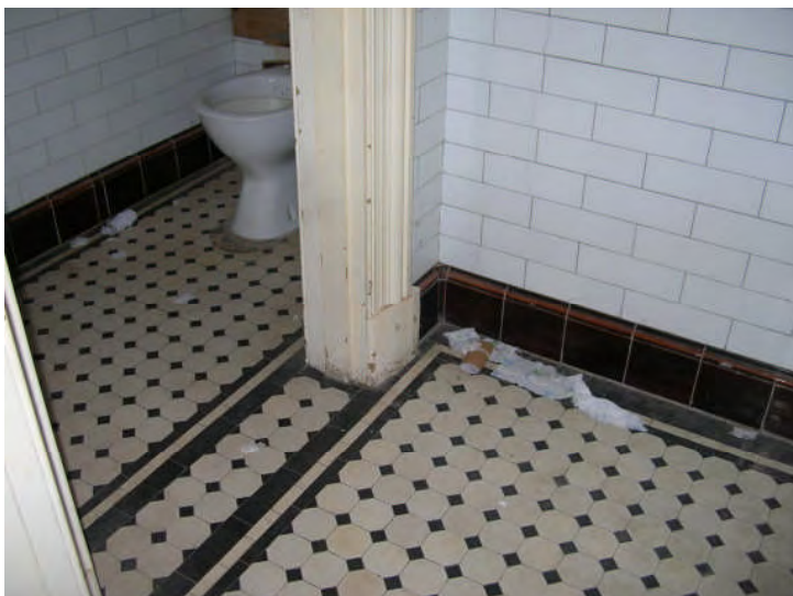
Figure 97 Tiled floor in vestibule and toilet.
