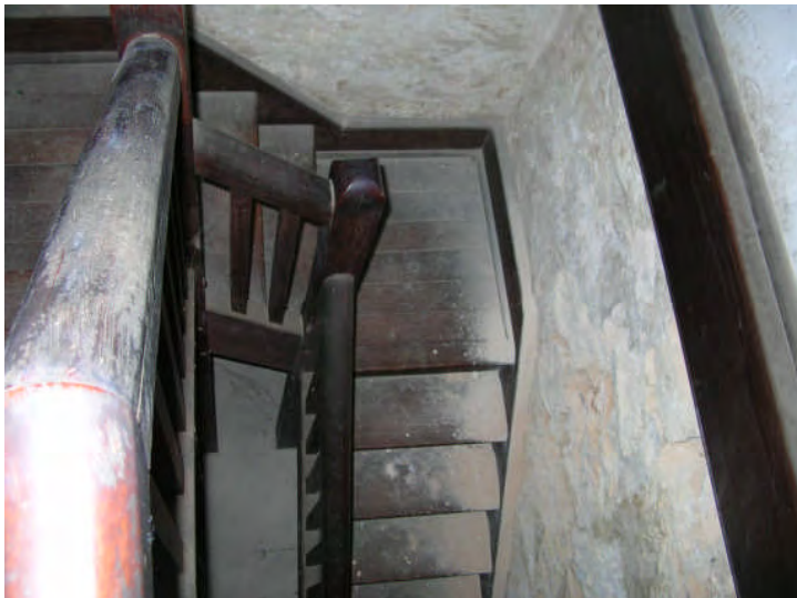
Figure 96 Stairs to cellar.
