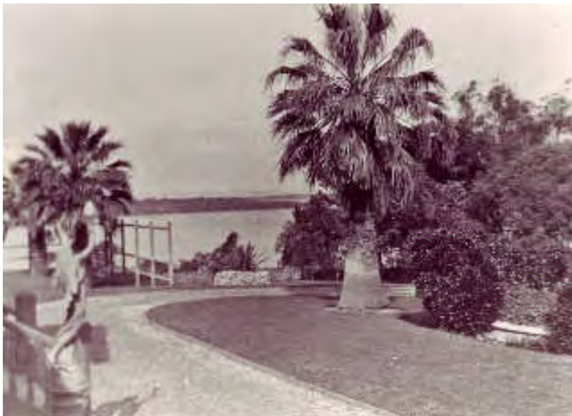
Figure 20 View of The Cliffe Grounds, 1920s. Courtesy of PLC archives
