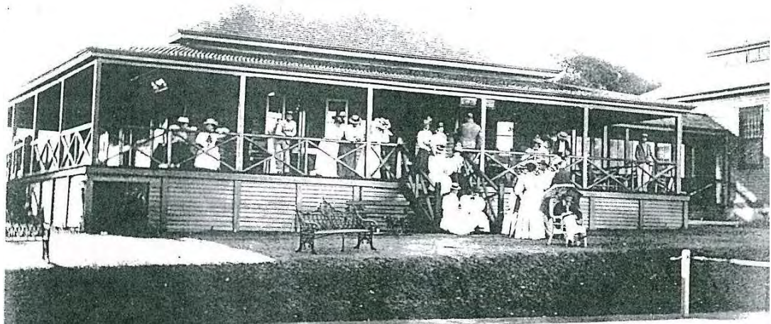
Figure 1 Historical Image of The Cliffe. Image Courtesy Battye Library 5395B/6.
