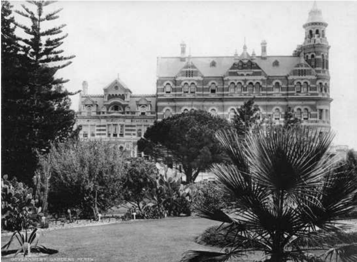
Figure 108 McNeil Chambers, Barrack St at left. (Demolished)
