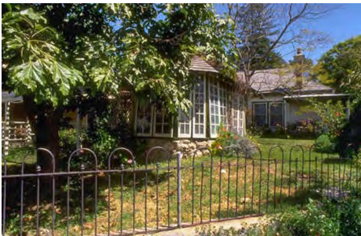
Figure 30 View of The Cliffe taken September 1995, for Register of National Estate.
