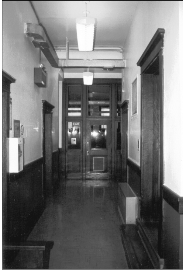
Plate 10 – Cornish Library, 20 West Gate, basement. ( M. Peterson, 1992. )
