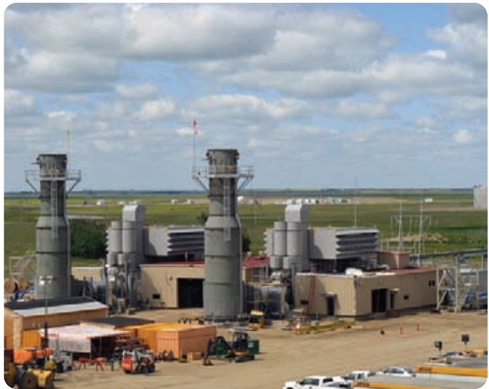
Located near Kerrobert, SaskPower's newly-constructed Ermine Power Station has a capacity of 92 MW from two natural gas-fired units. Gas-fired plants can be constructed quickly and economically, and are helping to reinforce our company's system so that more wind generation can be added.
