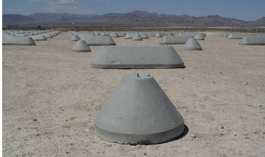
Figure 27: T20 pre-cast foundations in field installation
