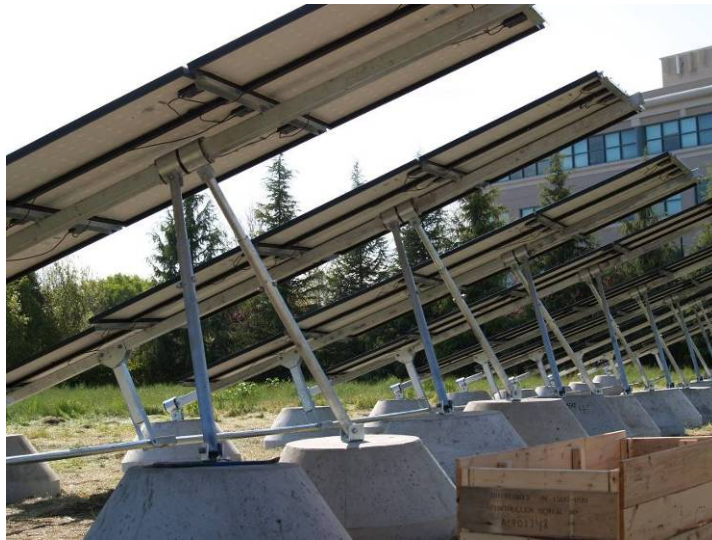
Figure 29: Telescoping legs allow for efficient stacking for transportation and quick installation.
