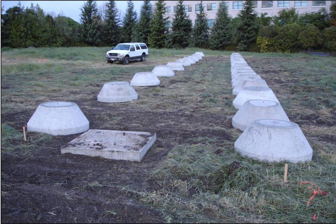
Figure 40: Installed Foundations.
