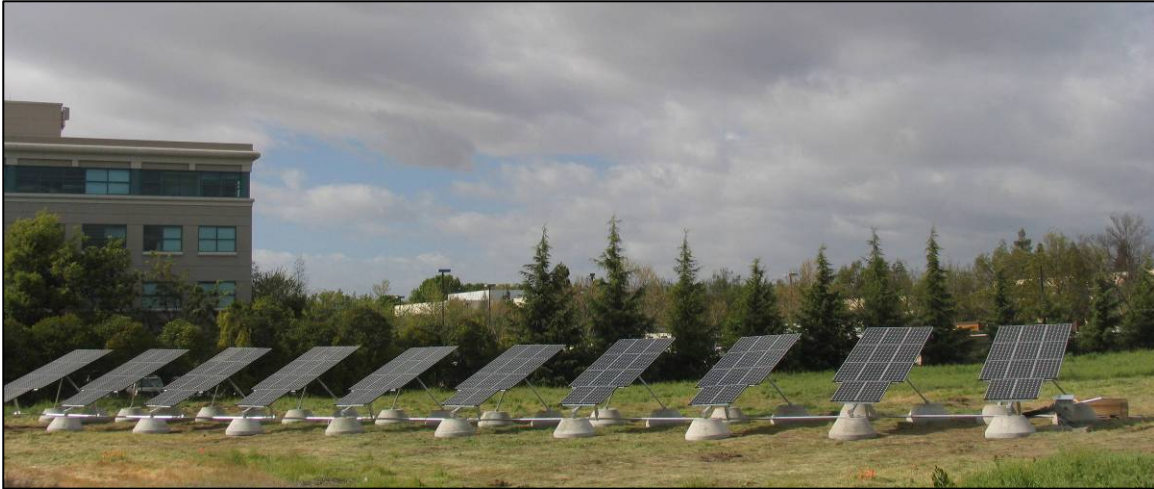
Figure 41: 10-unit demonstration installation
