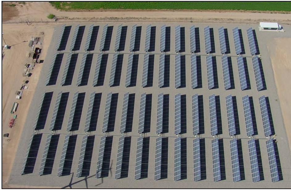
Figure 25: T0 ground system installation, including two drive units.
