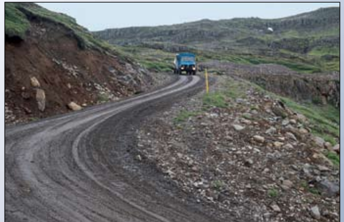
Mjóafjardarvegur (953), secondary road.
