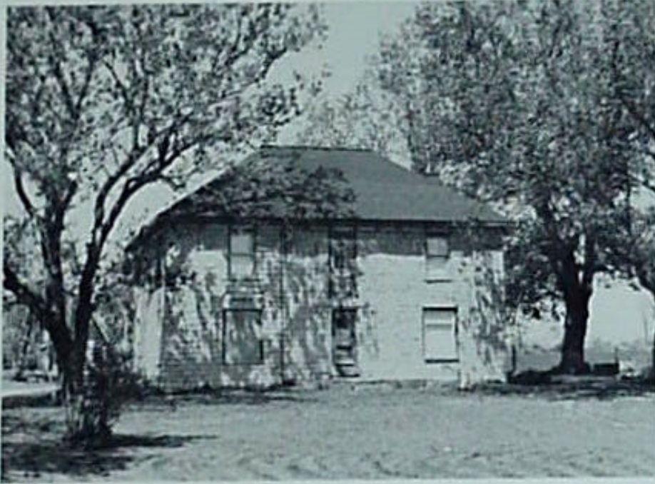
Arthur Farm First two-story stone house in Storrington Township ~ see page 167
