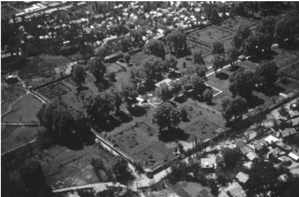
13. Aerial view of Shalimar garden, Kashmir (photo: courtesy of Michael Brand)
