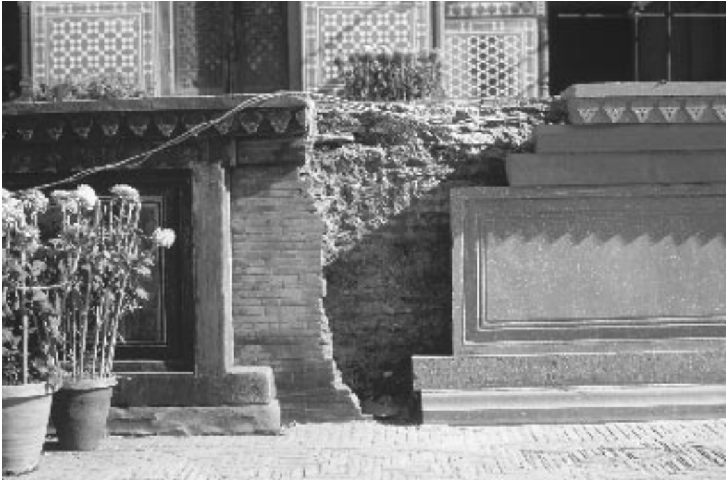
8. Layers of partially documented conservation work on the plinth of Jahangir's tomb-garden, Lahore, Pakistan
