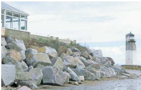
Coastal defences at Southerness
