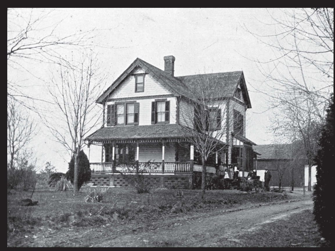
The George Crossman House from Charles Stewart's A Virginia Village , 1904. The house is located on N. Underwood Street. It is a local Arlington historic district and on the National Register of Historic Places
