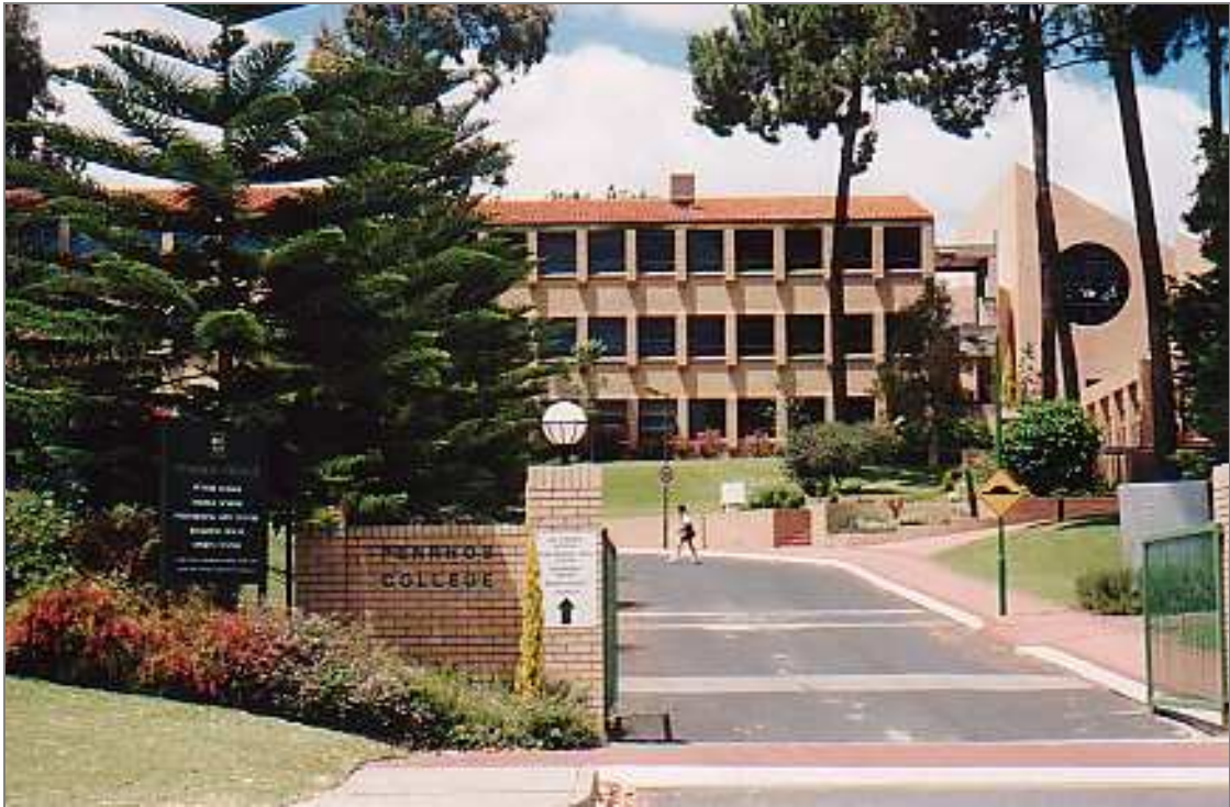
Entry to Senior School and Performing Arts Centre (note the Chapel on the right in background). (Heritage TODAY 1999)
