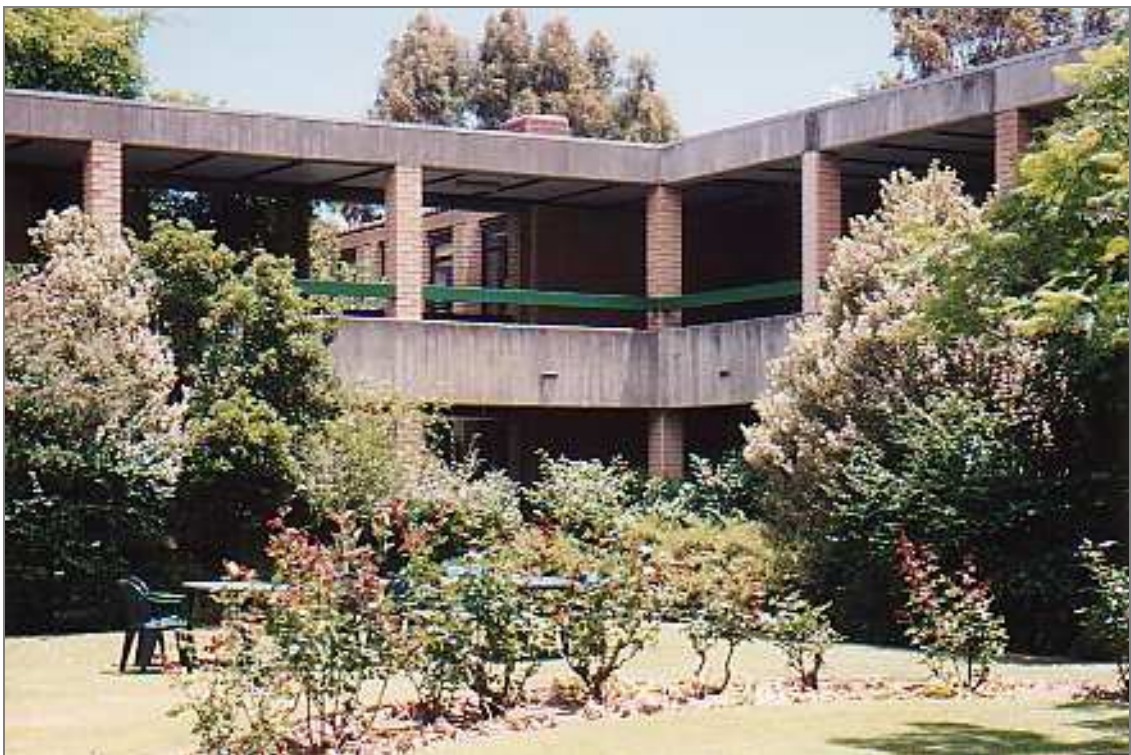
One of the original classroom blocks now Science Department and Staffroom. (Heritage TODAY 1999)
