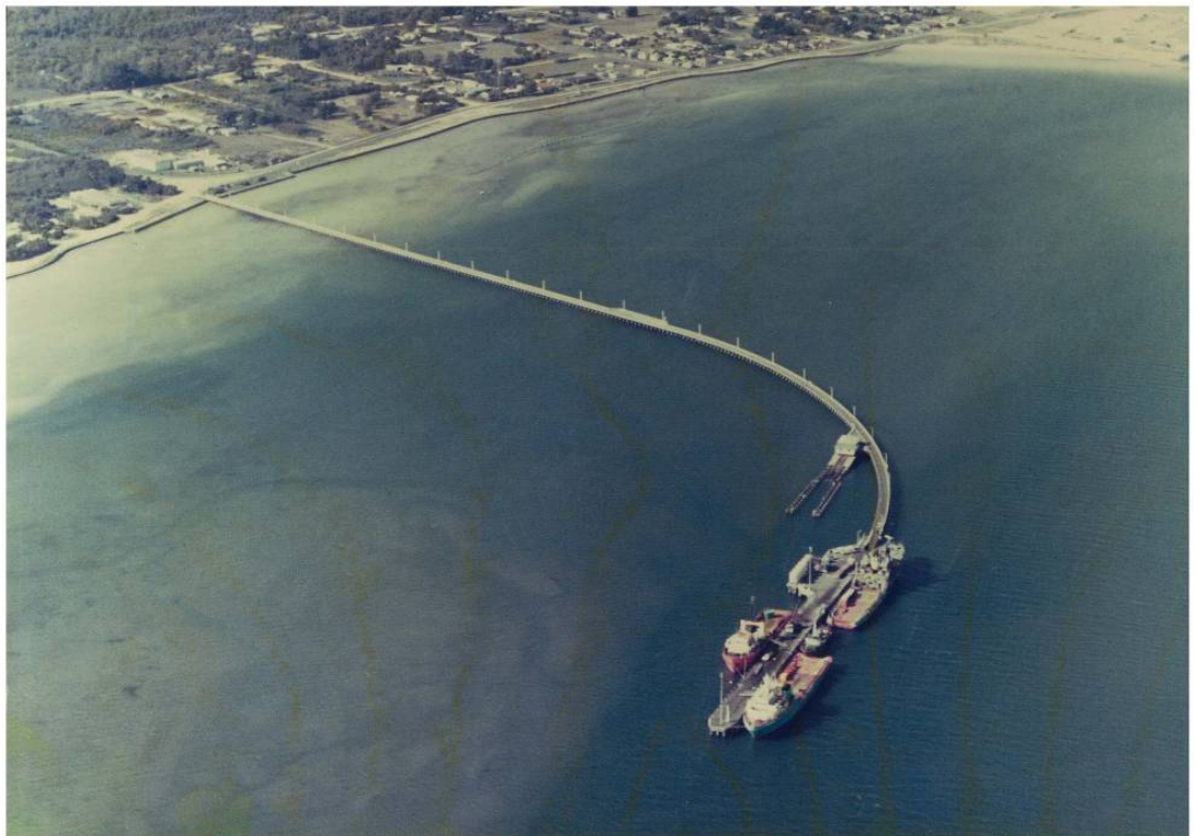
Figure 1: The Long Jetty at the height of its use for the oil industry in the mid 1980s.
