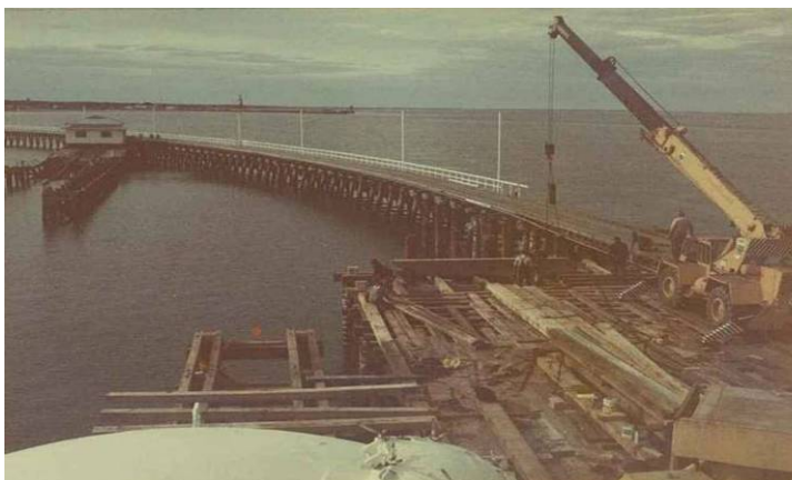
Figure 21: Hornibrook's Construction of the extended turning bay in 1982.
