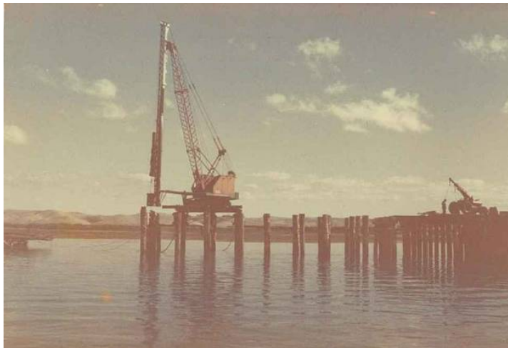
Figure 39: The 60m extension under construction in 1982.
