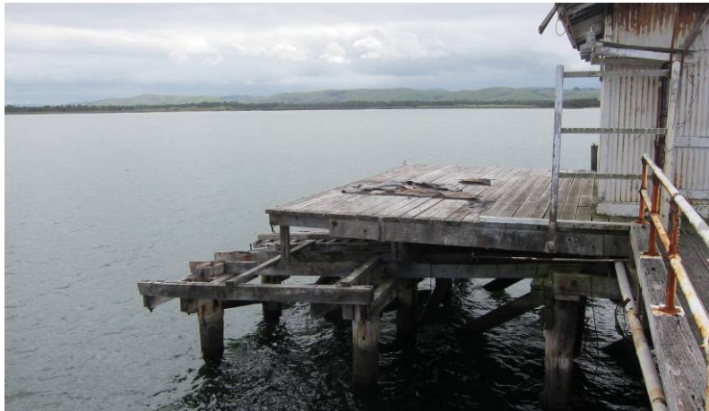
Figure 29: Truncated remains of the slipway to the rear of the slipway shed.
