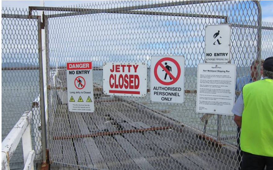
Figure 24: Gates erected across the jetty approach.
