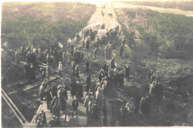
Figure 6: The view looking north at the Midland Highway. Norry Rossitter stands on the pile driver to take this photo (photo source: Norry Rossitter).
