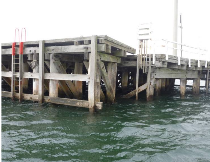
Figure 38: The 1982 tank stand, raised above the adjacent turning bay.
