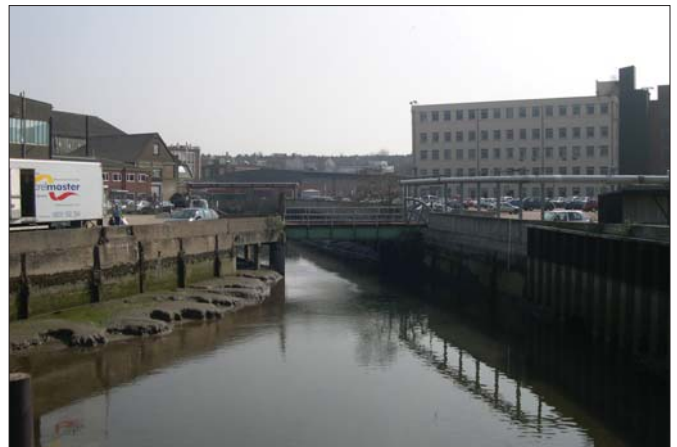
View north back into town from Dartford Creek
