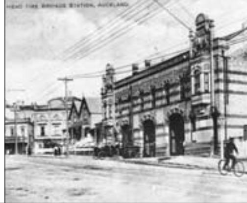
35. Head Fire Brigade Station | 50 Pitt Street
