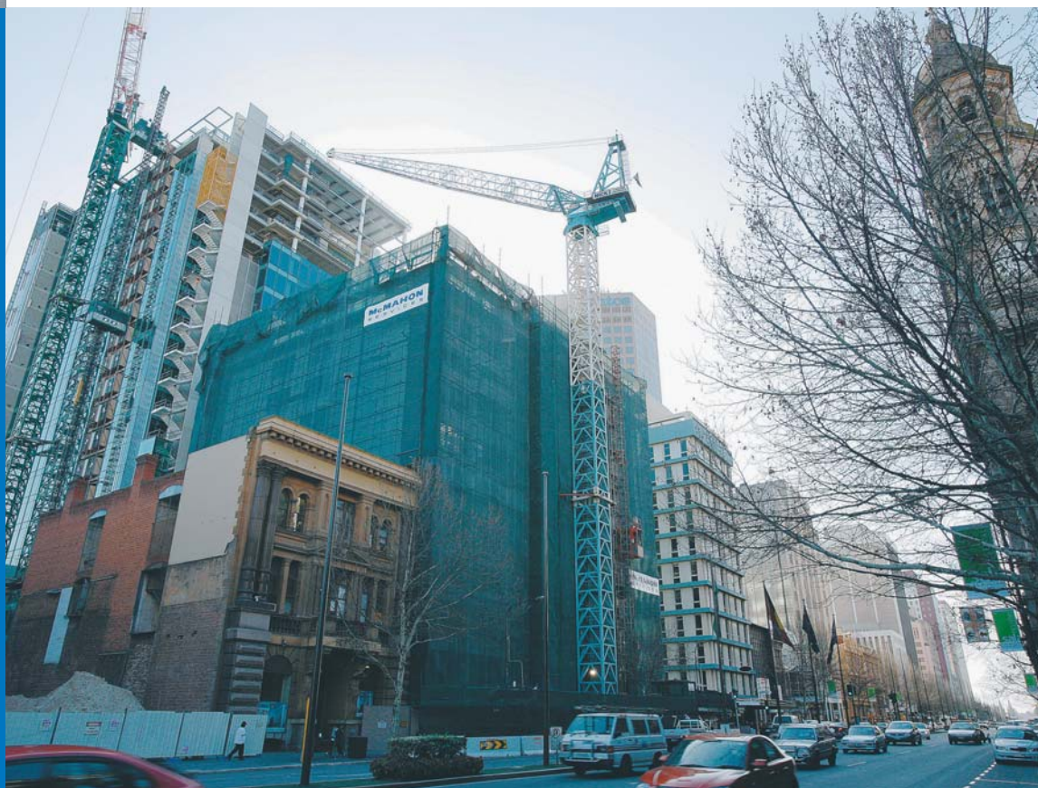
Major development on King William Street
