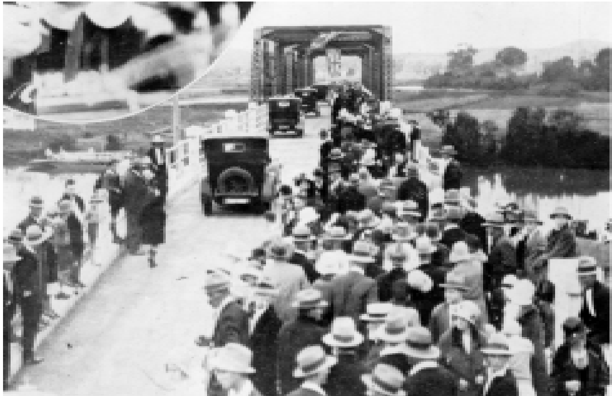
Opening Loganholme Bridge 1931 (Source: The Queenslander)
