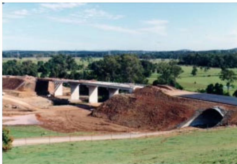
Building Logan Motorway (Source: Logan City Council Collection)
