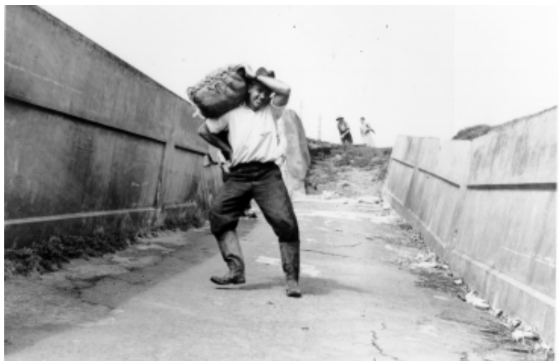
The high sides of the narrow Waterford Bridge which gave it the nickname “The Pig Trough” are obvious in this photograph. George Fredericks is carrying a bag of potatoes down the tilted surface of the bridge after the 1947 floods. (Source: Joan Starr)
