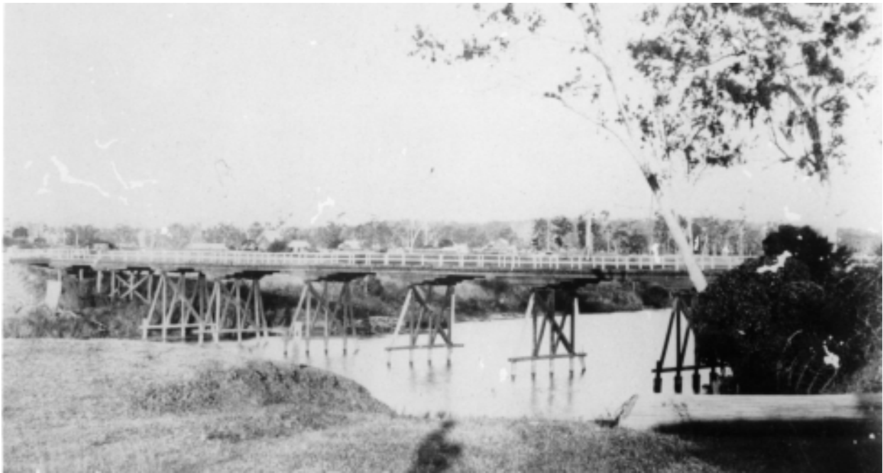
Waterford Bridge in the 1880s. The bridge had a somewhat experimental design with long 50ft spans and light planking
