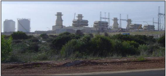
Figure 1: Ankerlig OCGT power station (four OCGT units and two fuel tanks are shown)
