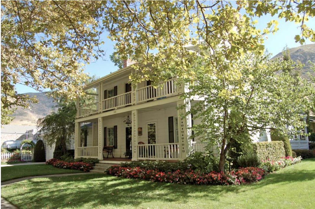
Photograph 5. Hector Haight House/Union Hotel. 208 North Main Street. Camera facing northeast.
