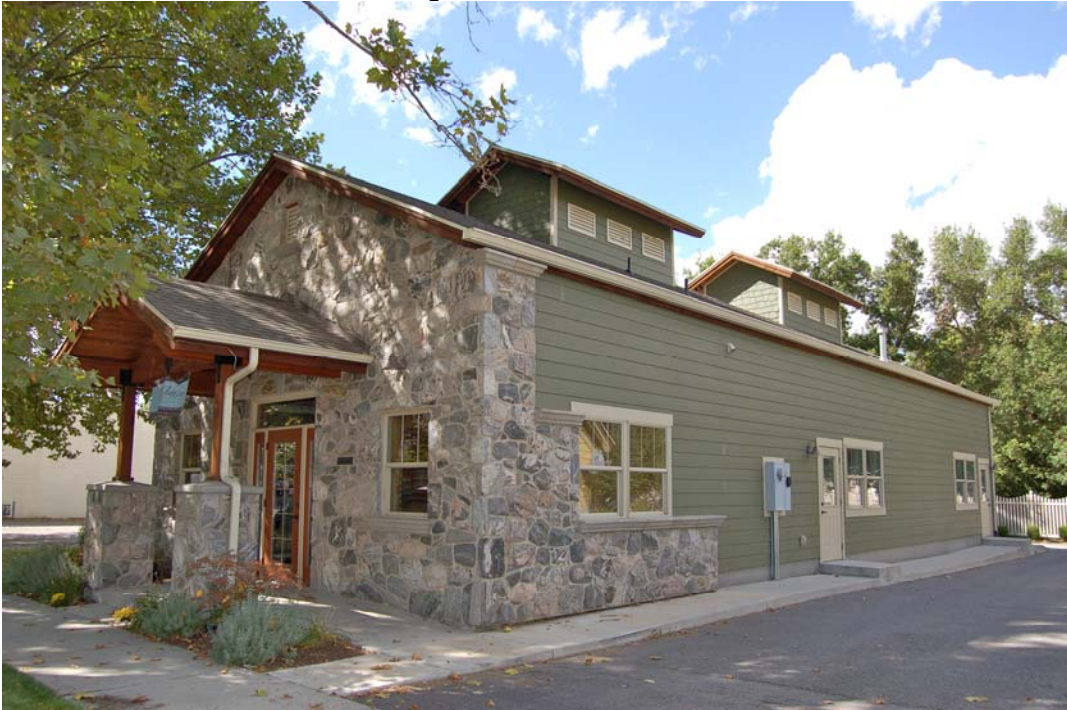
Photograph 24. 63 North Main Street. Camera facing southwest.
