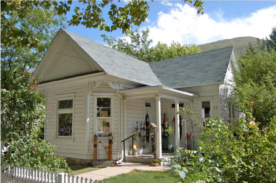
Photograph 18. 58 North Main Street. Camera facing northeast.
