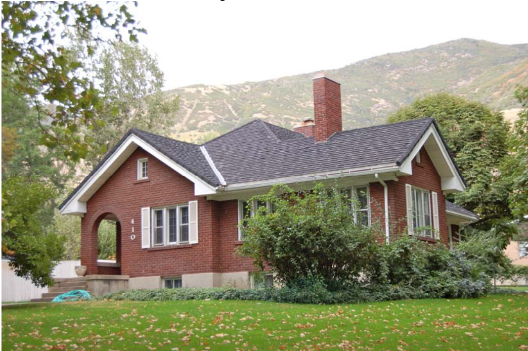
Photograph 21. 410 North Main Street. Camera facing northeast.
