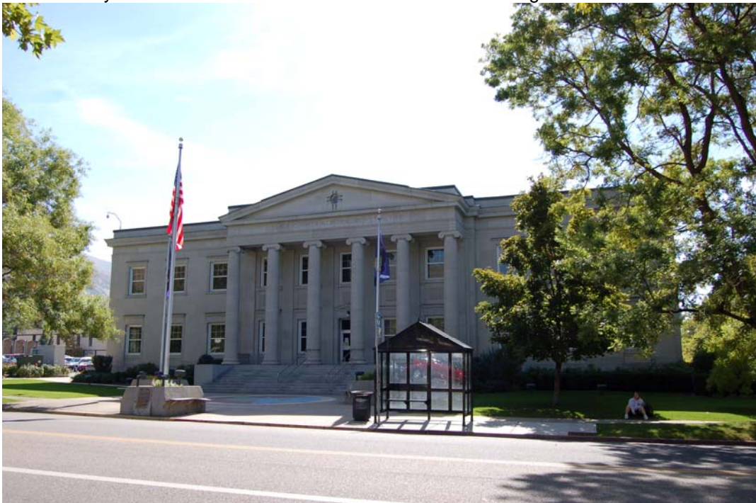
Photograph 15. Davis County Courthouse. 28 East State Street. Camera facing southeast.
