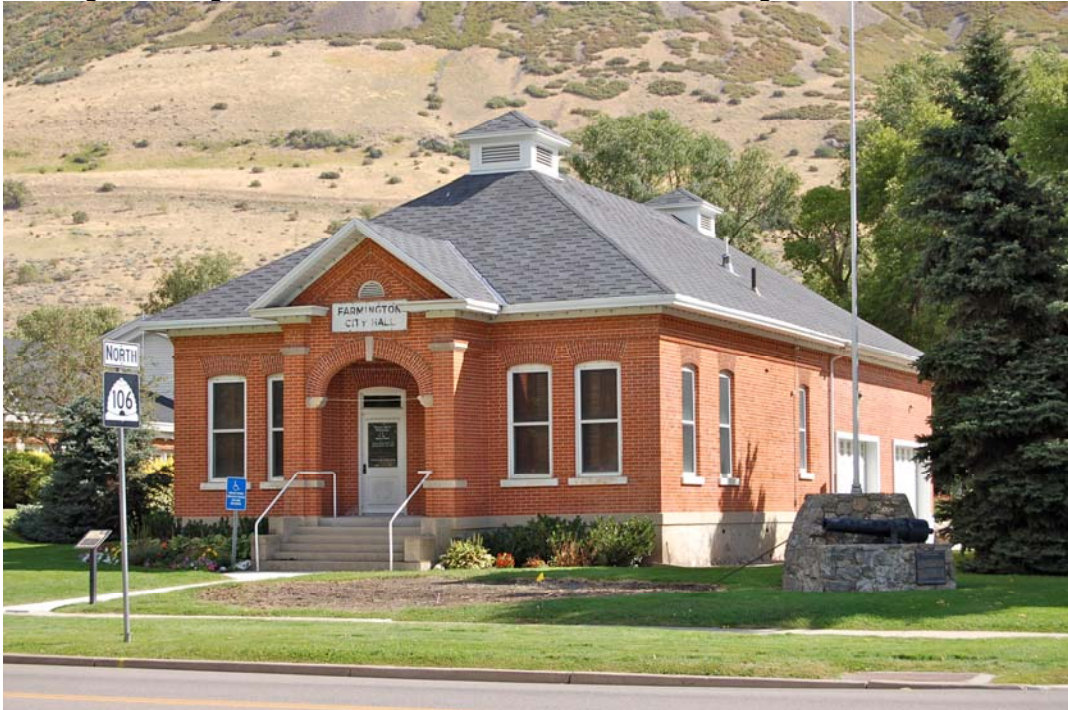
Photograph 14. Farmington Tithing Office. 108 North Main Street. Camera facing northeast.
