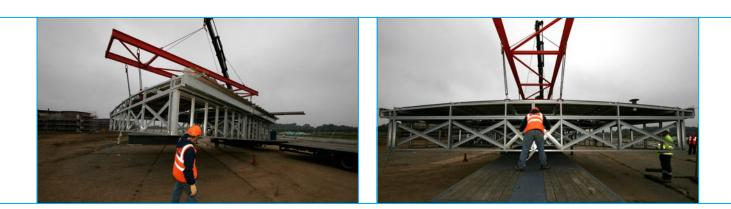
At Marne, the modular roof units were assembled on a disused runway. These roofing sections were purposebuilt for the Marne project. Once the main building frame had been constructed by a modular building specialist, the entire roof structure was lifted and secured in place. Eight modular roofing sections were fitted on to each building – two for the central core, and two for each of the three wings.
