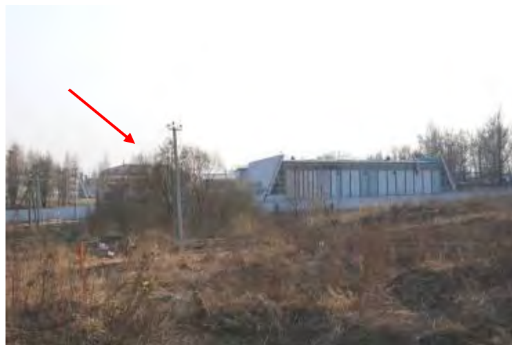
Fig. 9. Severed power cables (item 7 fig. 2)
