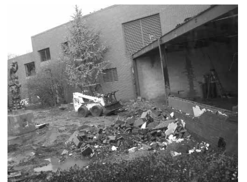
Demolition of Warshauer Quiet Lounge
