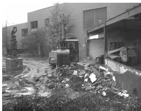
First phase of Courtyard demolition
