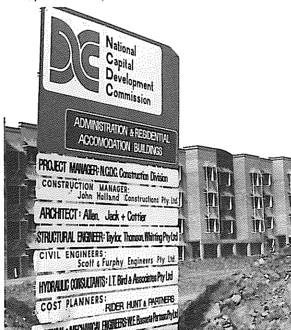
Halls of Residence, AIS, under construction (Architects: Allen, Jack and Cottier)
