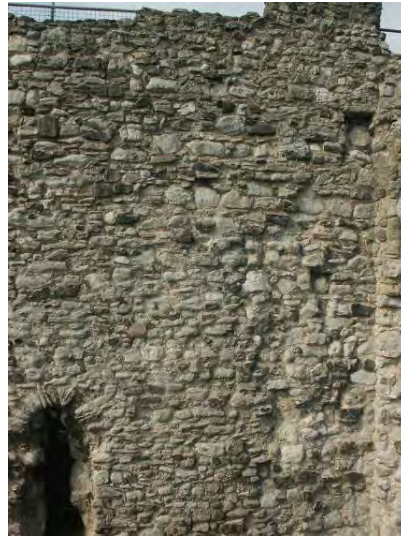
E elevation, remains of window jamb
