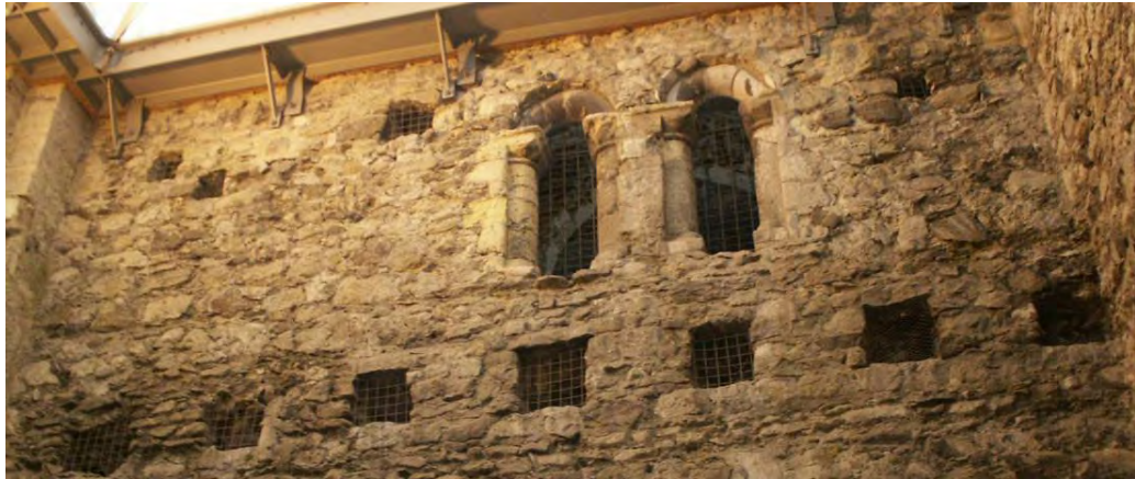
Forebuilding, window blocked during medieval period
