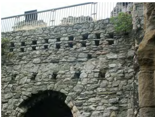
North elevation, detail of rafter sockets and pigeon holes
