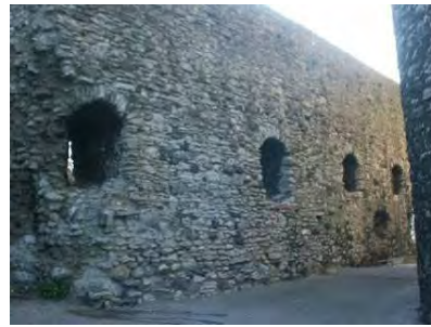
South curtain wall, interior
