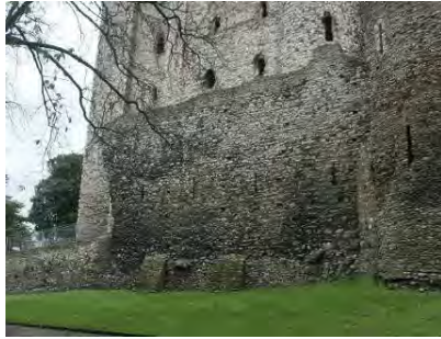
South curtain wall, exterior
