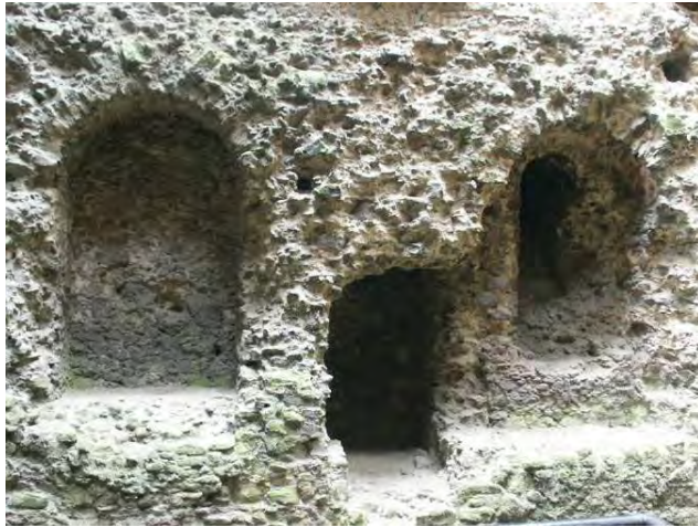
Basement south elevation, remains of rectangular opening
