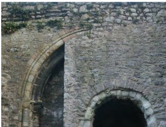
Third floor southern compartment, blocked arch
