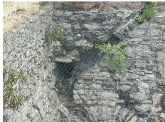
Northern compartment, east wall, roof scar
