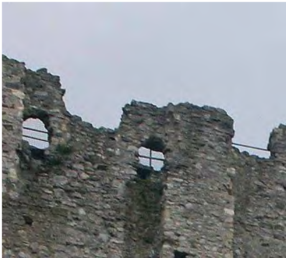
N elevation, entrance to brattice
