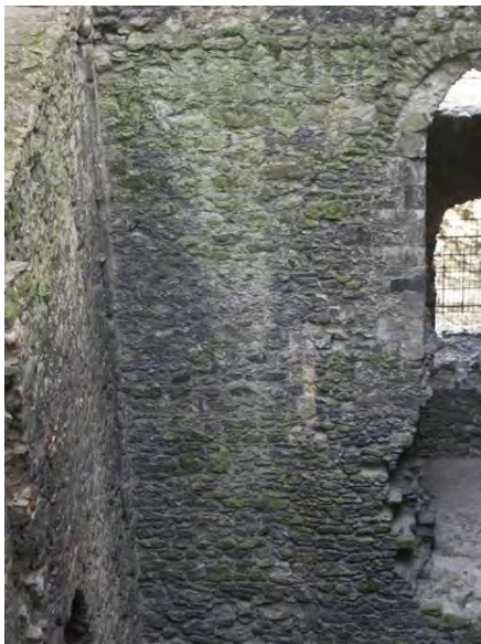
First floor, east side: quoining of blocked archway
