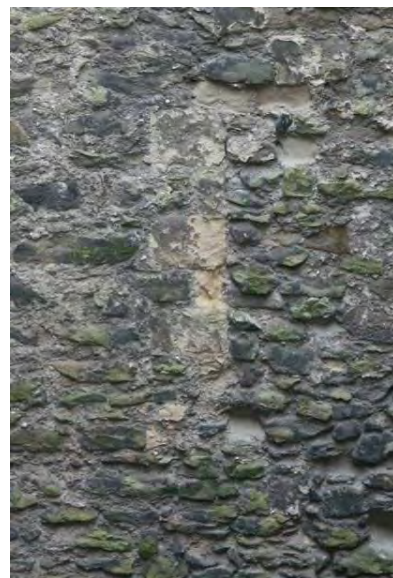
Detail of quoining
