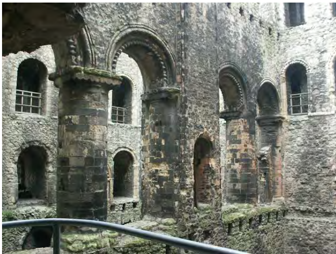
Second floor: arcade
