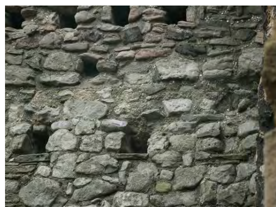
North elevation, detail of rafter sockets
