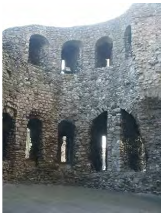
Drum Tower (Tower One), interior
