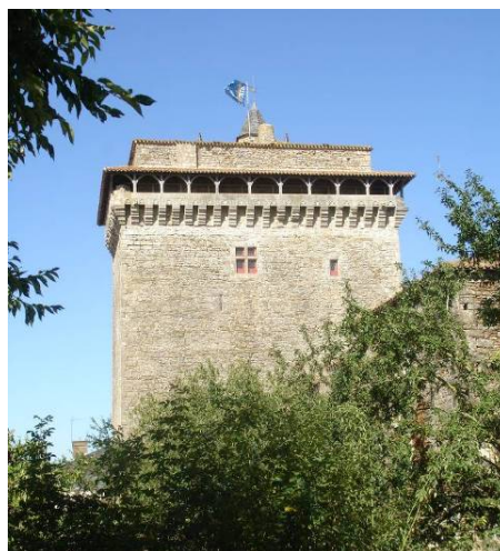
Re-roofed donjon at Bazoges
