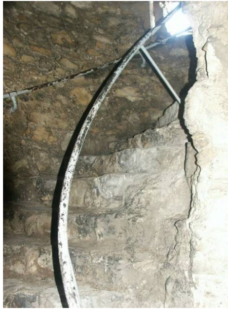
Current condition of north-east stair
