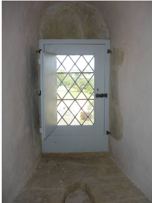
Bazoges, reinstated window opening
