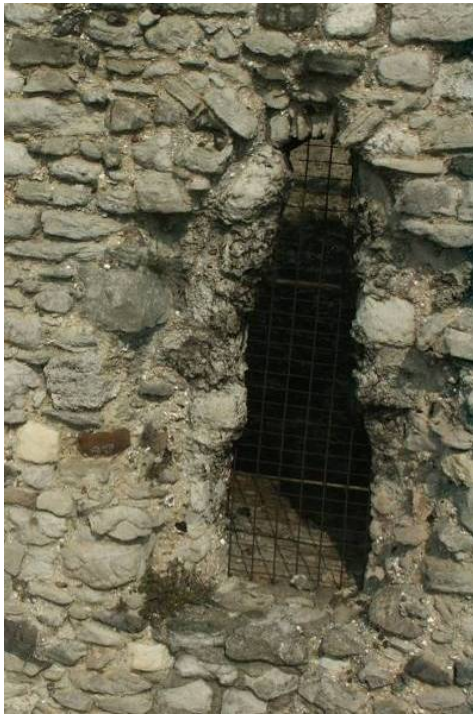
South elevation: complete window opening
