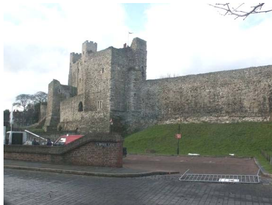
The car park
