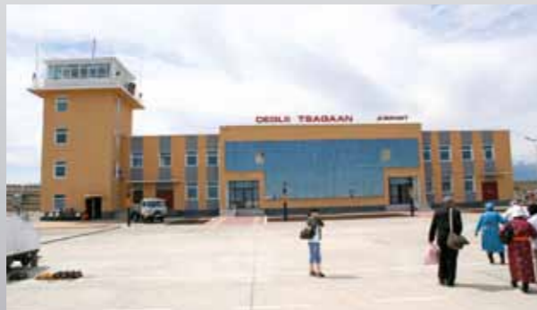
The terminal building at Ulaanbaatar has undergone recent renovation.
