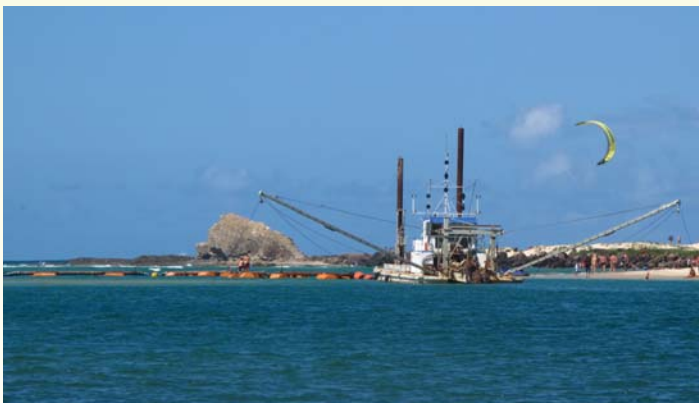
Dredge in Currumbin Creek (Source: GCCC)
