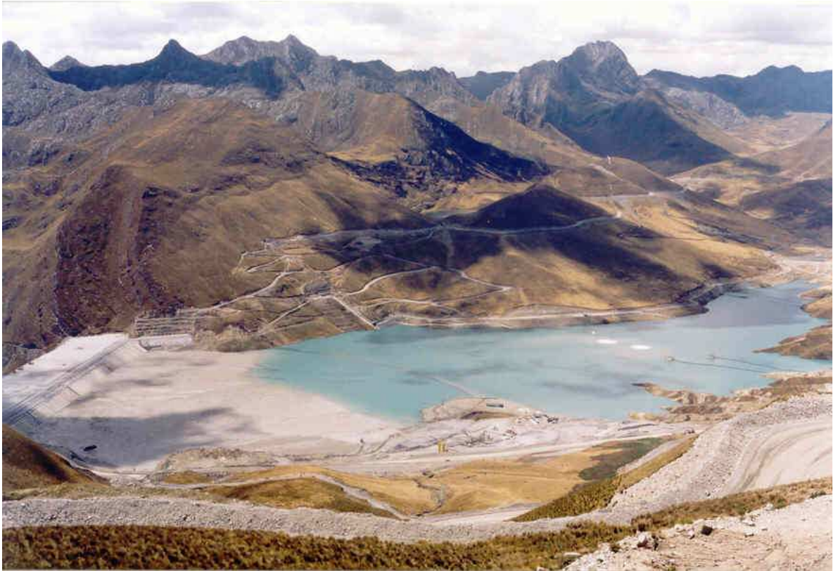
Figure 3 Tailings Impoundment Facility: September 2002
