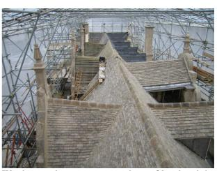
We then made our way up to the roof level and the lead flats behind the parapet. The access gantry across the roof gave a fine view of the roof slating in progress.
