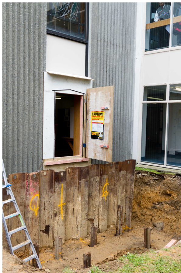
Piles being installed for the foundations of the new lift which will go outside the staffroom.
