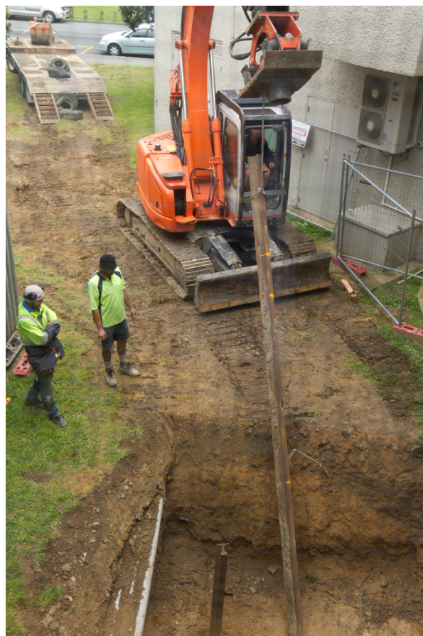
Piles being installed for the foundations of the new lift which will go outside the staffroom.
