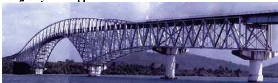
The San Juanico Bridge between Samar and Leyte Islands
