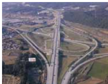
AH1 Hobeop Junction in Daejeon
