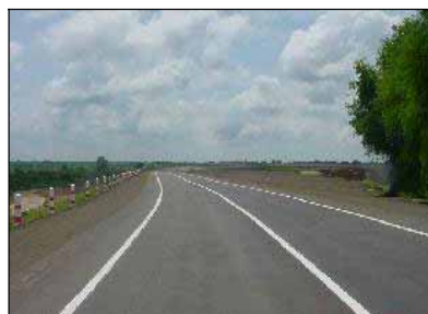
AH1: near Kizuma Bridge
