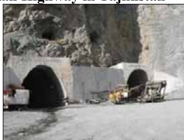
AH7: Anzob Tunnel Dushanbe to Anji
