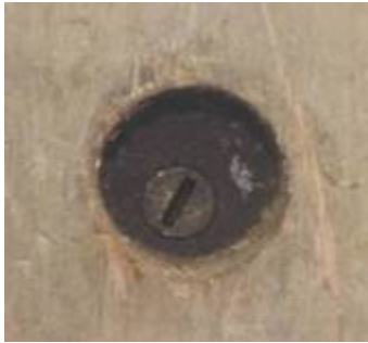
Lock Cylinder Removed
