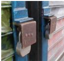
Welded Lock Cover
