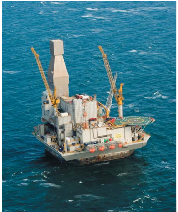
Drilling from the Orlan drilling and production platform commenced in December 2005, offshore Sakhalin Island.
