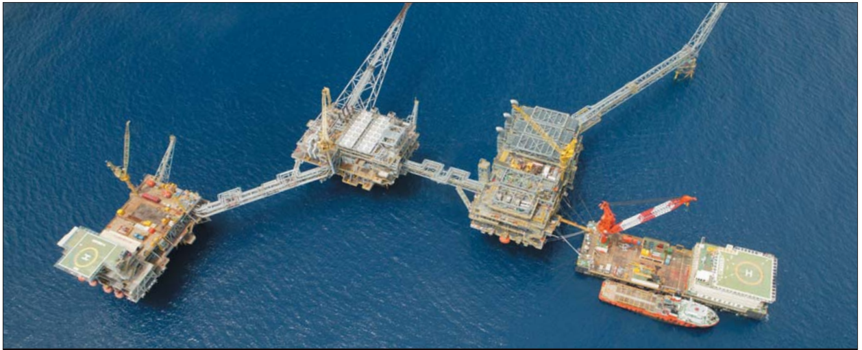
Guntong Compression Hub, offshore peninsular Malaysia. From left to right: Guntong D-Production, Guntong D-Compression, and Guntong E (under construction).
