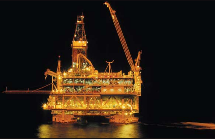
Production from the Kizomba A tension leg platform (above) is transferred to one of the world's largest FPSOs.
