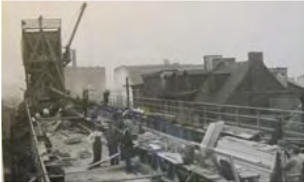
Construction of the elevated rail line along Front Street, 1917
