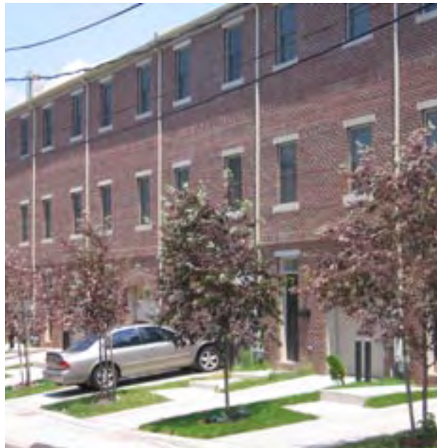
Streetscapes suffer from addition of garage doors.
