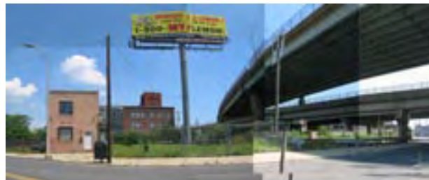
Existing condition of land below I-95 and the EI.
