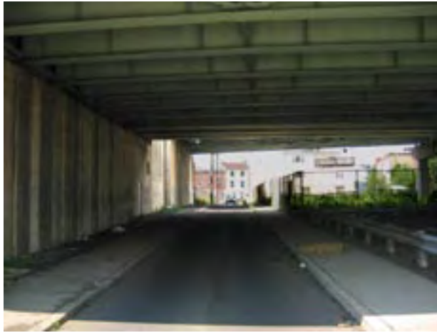
Existing Ellen Street underpass
