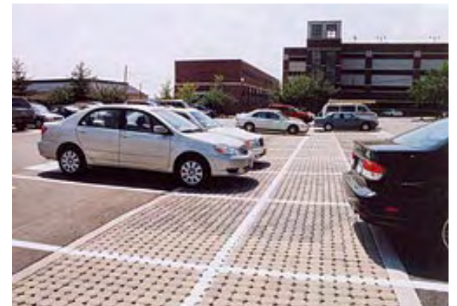
Top: Edge plantings to detain rainfall from buildings. Bottom: Permeable materials used for parking lot drainage.
