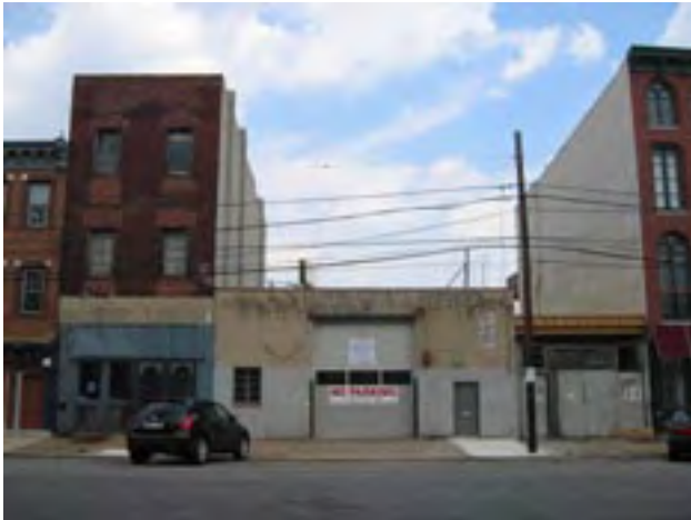
Loading docks along 2nd Street
