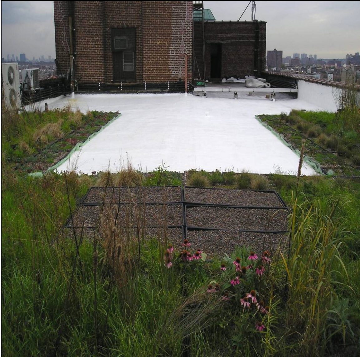
Figure 6. Modular Cool Roof and Green Roof System of Sustainable South Bronx's Smart Roof Demonstration Project
