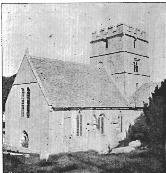
VIEW OF CHURCH FROM S.W.
