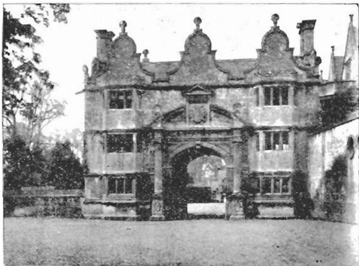
GATEHOUSE, STANWAY HOUSE.
