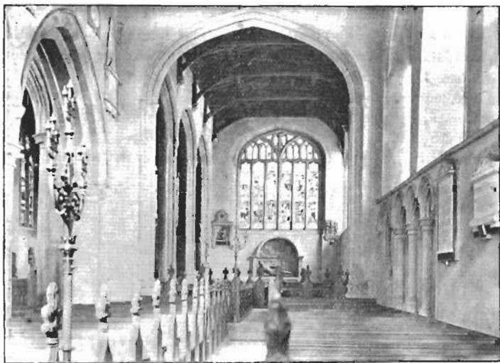
SOUTH AISLE, WESTBURY.
