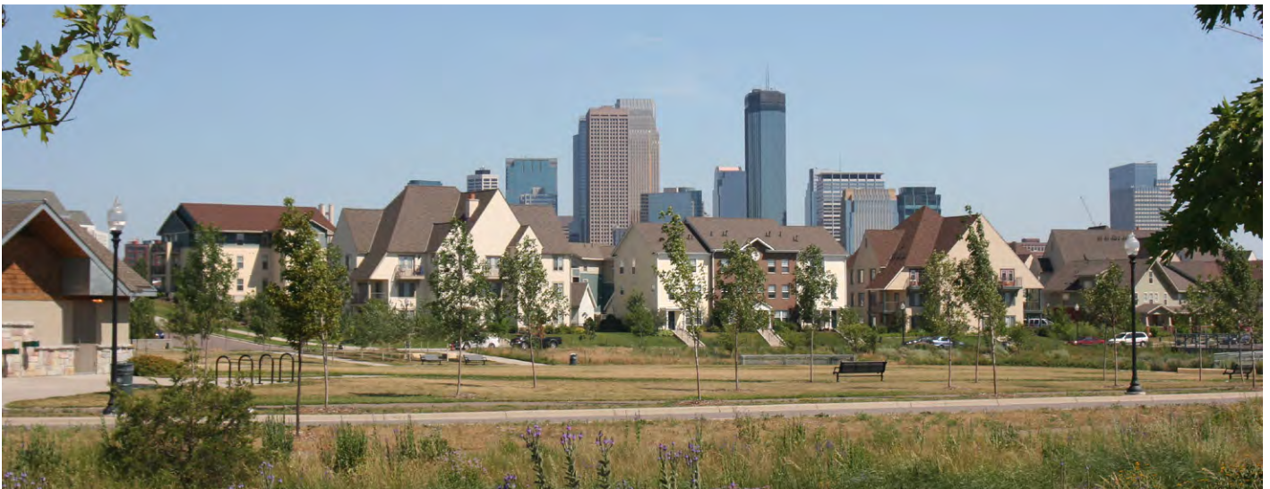
A continuum of housing styles and types ensures a vibrant mixed-income, multi-generational development at Heritage Park, Minneapolis, MN
