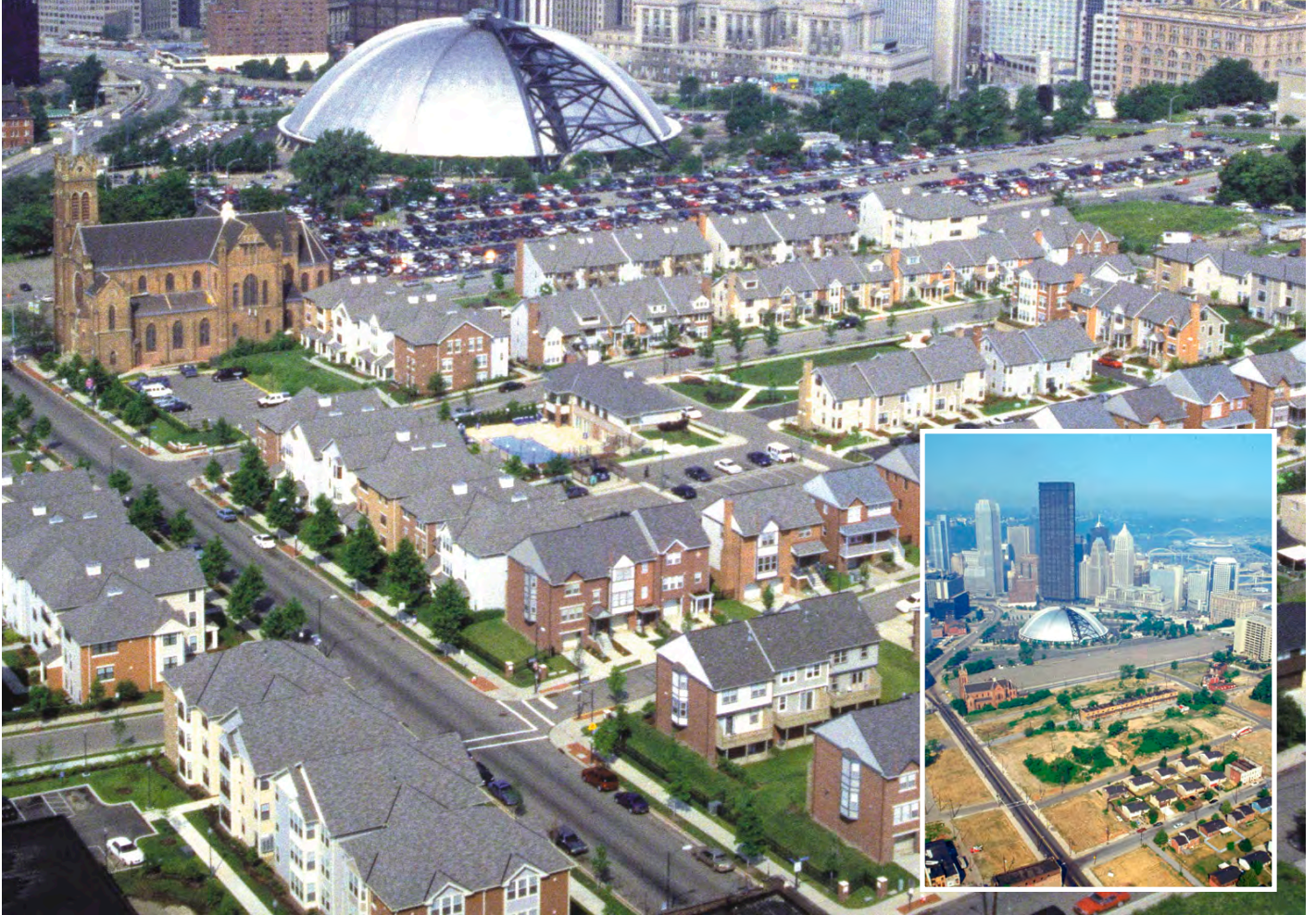
Crawford Square neighborhood revitalization in Pittsburgh, PA, both before (inset) and after.
