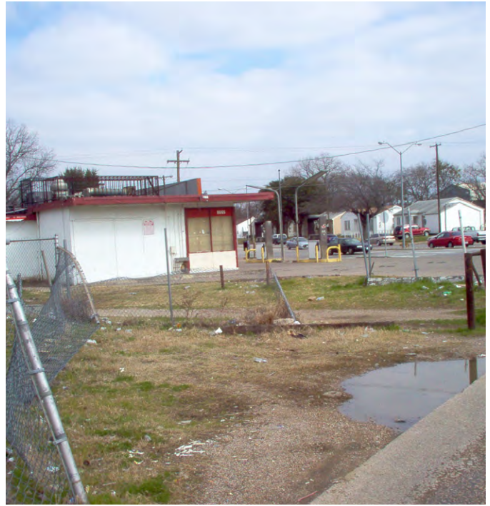
Distressed and abandoned property in Frazier Park, Dallas, TX
