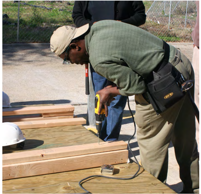
Community residents learn construction trades at Harmony Oaks, New Orleans, LA.
