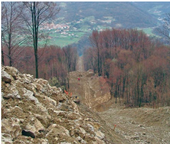
View along the alignment of the penstock
