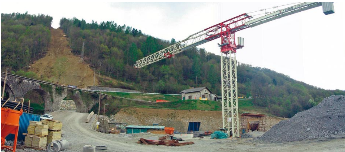
Construction of the powerhouse shaft, in the background soil excavation for the penstock
