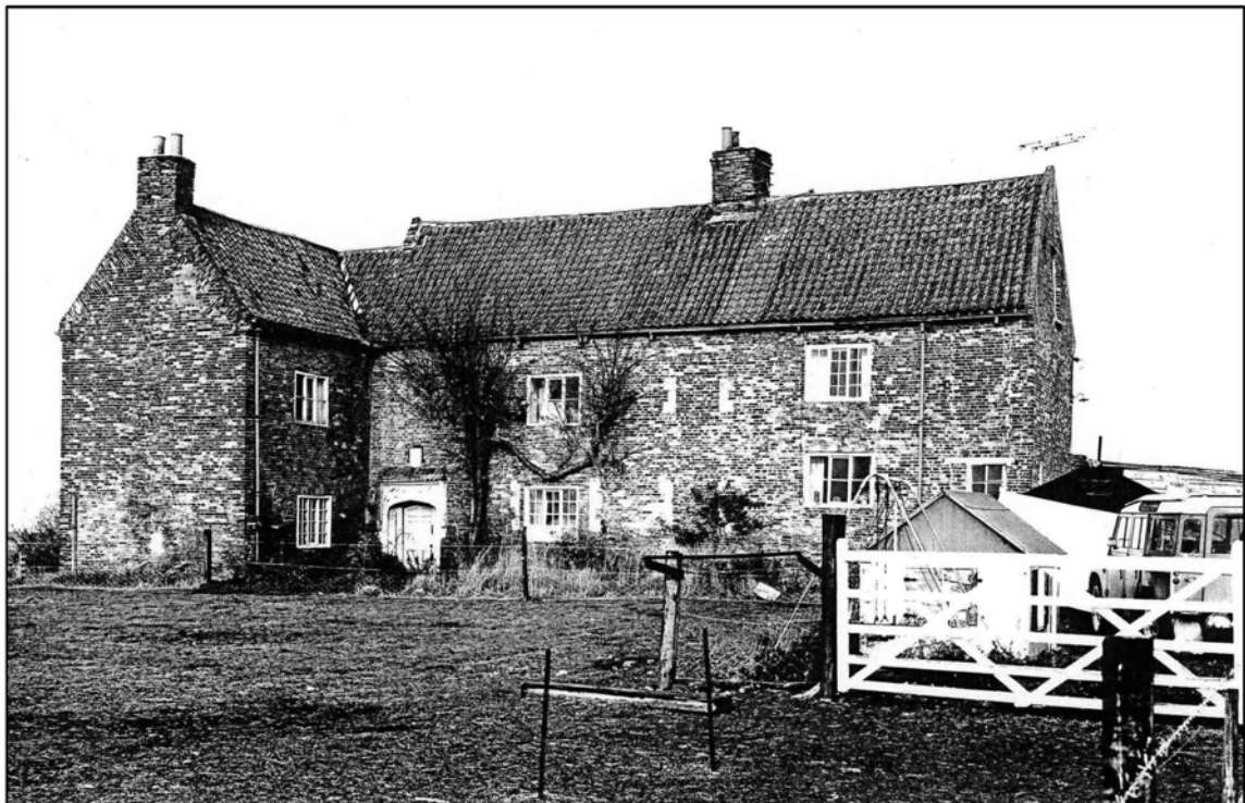
Plate 2: Haltemprice Priory farmhouse, looking north, November 1975 (© Crown copyright NMR BB77/7964)
