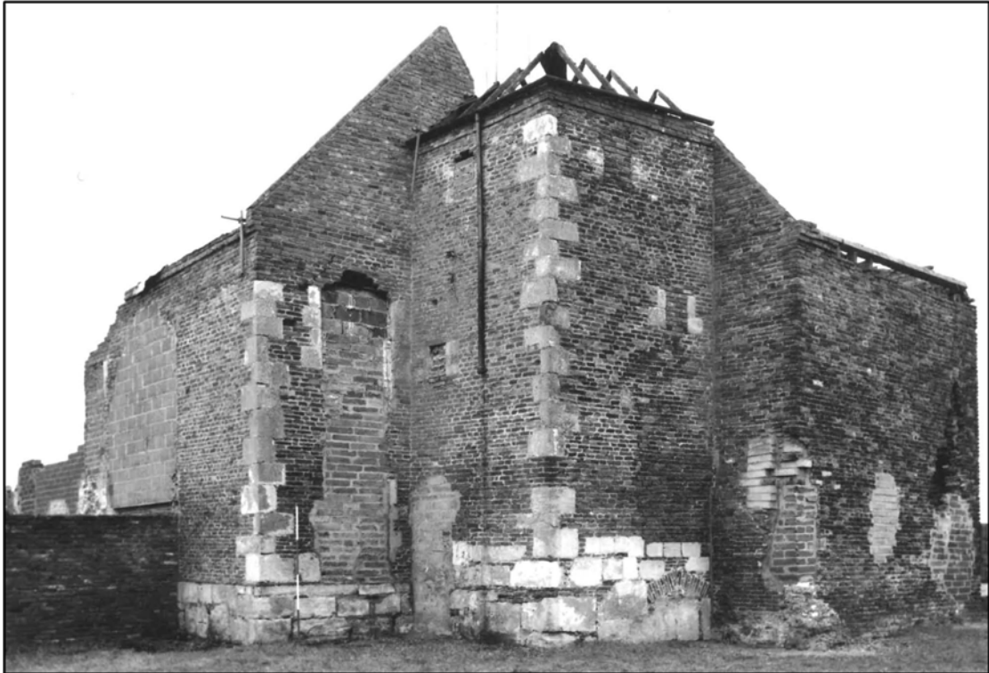
West side of farmhouse showing stair-tower, looking South-East, January 2004 (photo 1/8)
