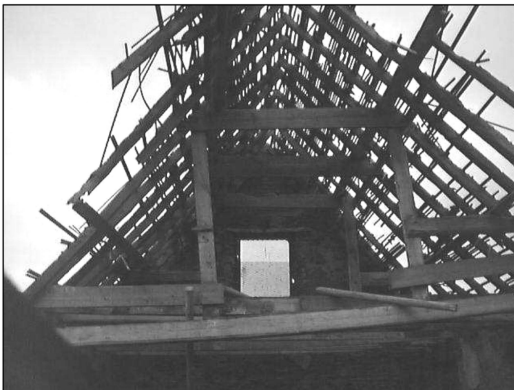
Plate 6: Roof structure over main range, c.2000 (Hadgraft collection)
