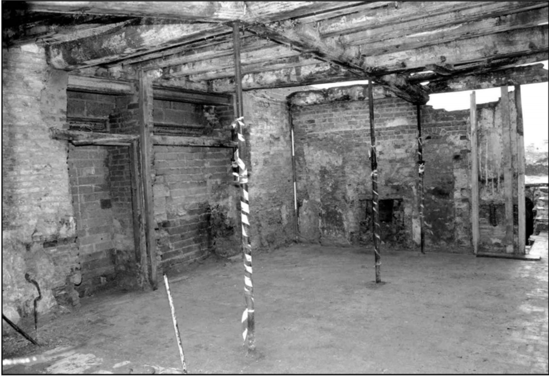
Plate 17: Ground floor main room after clearance, showing fireplaces in north and east walls, looking north-east, February 2004 (photo 3/17)
