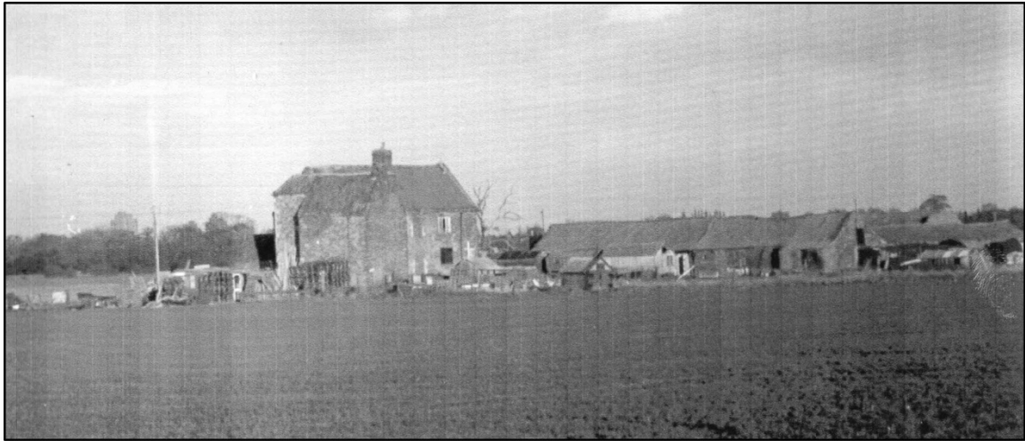
Plate 3: View of farmhouse and adjacent farm buildings, looking north-east, early 1989 (Hadgraft collection)
