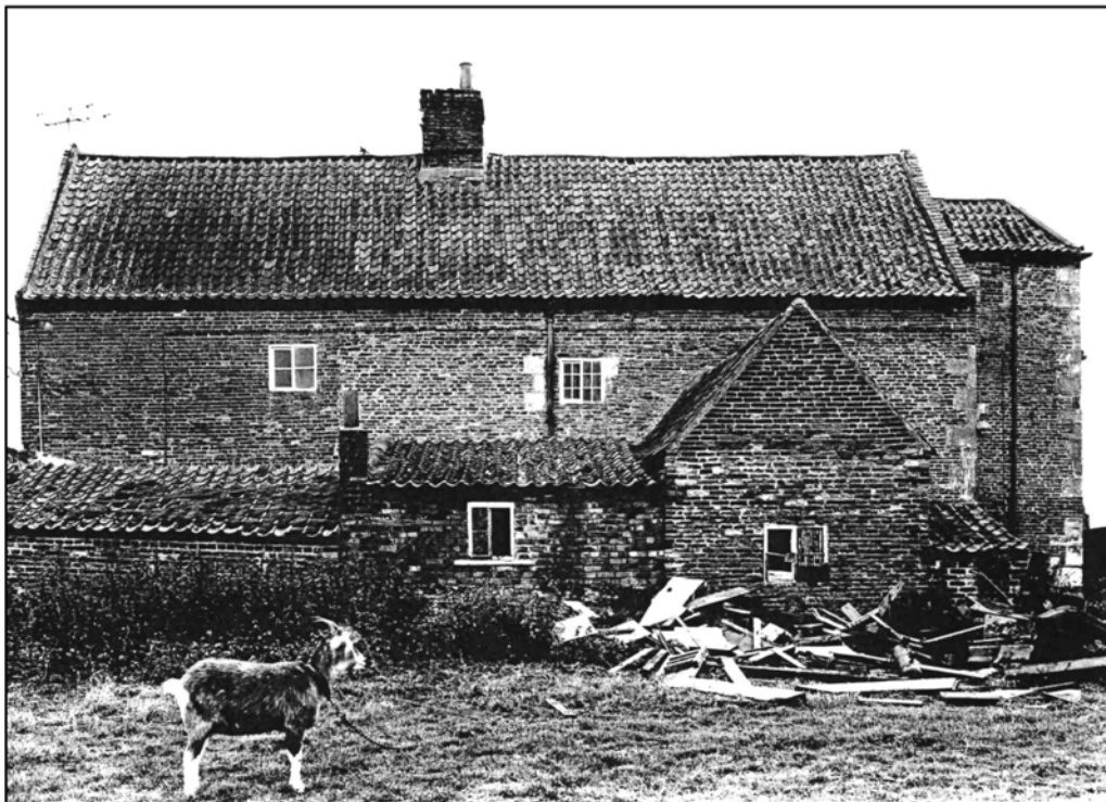
Plate 12: North side of farmhouse, looking south, November 1975 (© Crown Copyright NMR BB77/7969)
