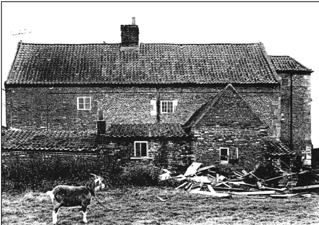
North side of farmhouse, looking South, November 1975 (© Crown Copyright NMR BB77/7969)
