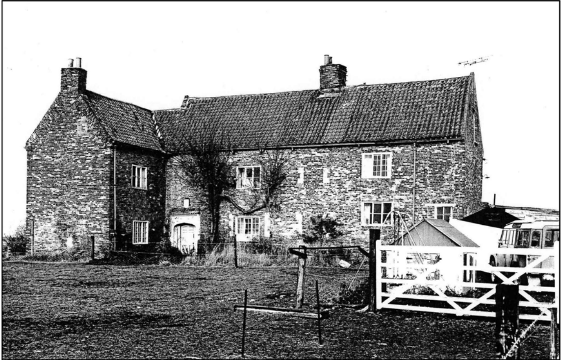
Haltemprice Priory farmhouse, looking North, November 1975 (© Crown copyright NMR BBBB77/7964)
