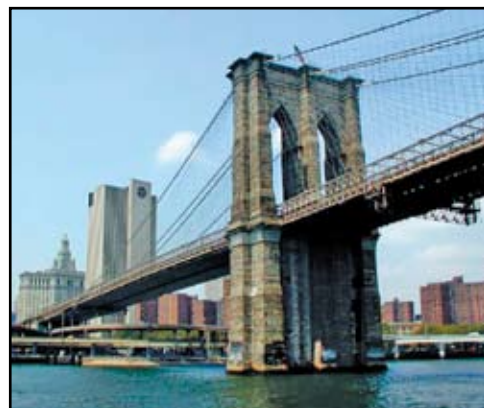
Brooklyn Bridge (Courtesy of HAER)
