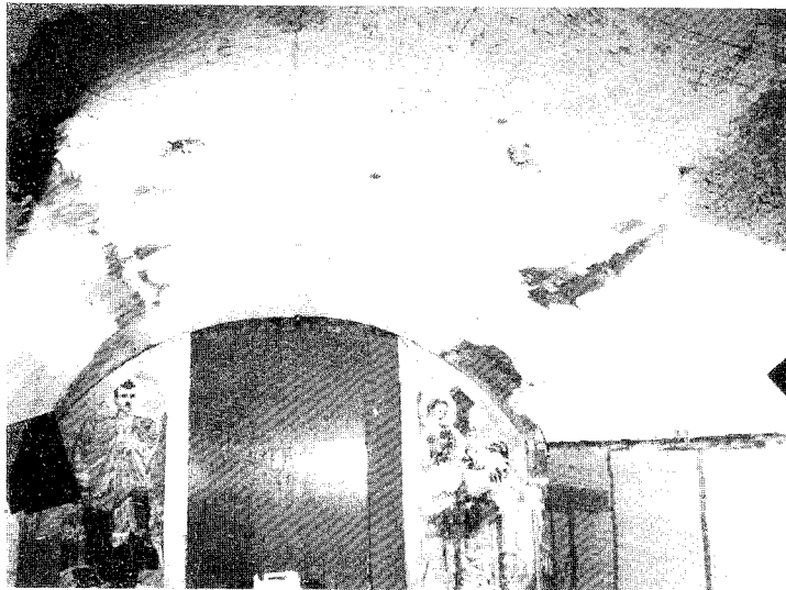
ILLUSTRATION IV During conservation Vaulted ceiling after mural removal. Visible original lime render and left fragments of gilded background.
