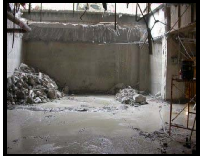
East Vault Demo, Top & West Wall
