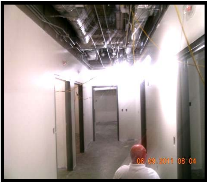
Painted Sheetrock Corridor
