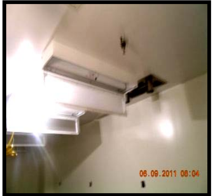
Ceilings and Walls painted, light figures being installed
