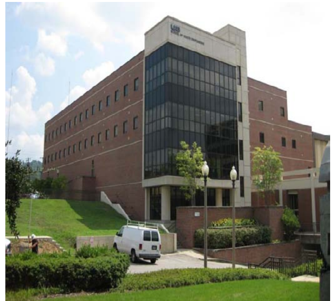
Addition of Two Floors - School of Health Professions Building
