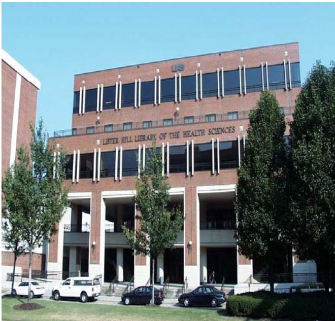
Fit-up, 4th FI - Lister Hill Library of the Health Sciences for Faculty Office Space
