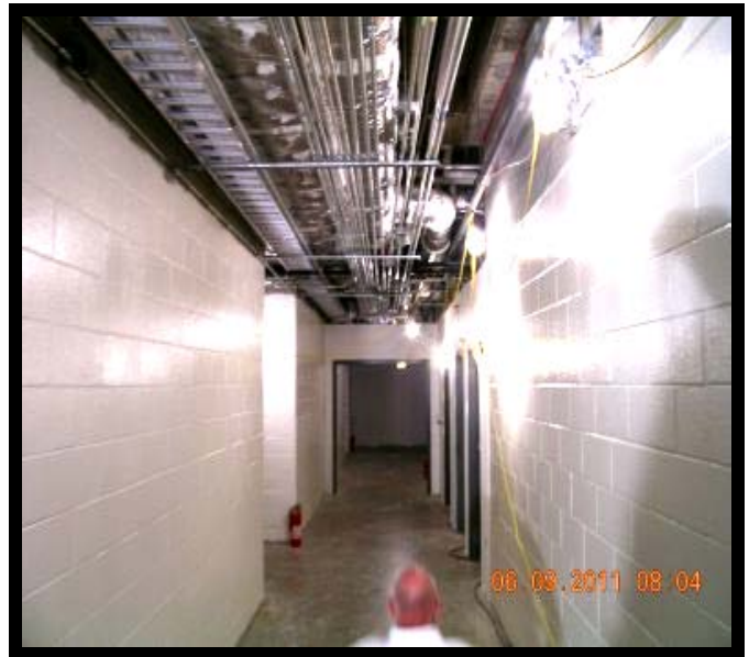
Painted CMU Corridor
