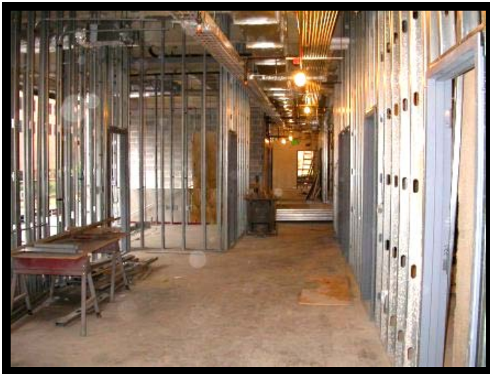
Wall Framing, 2 nd Floor
