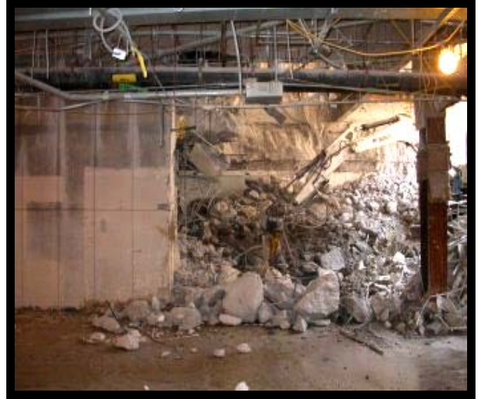
North Vault Demo In Progress
