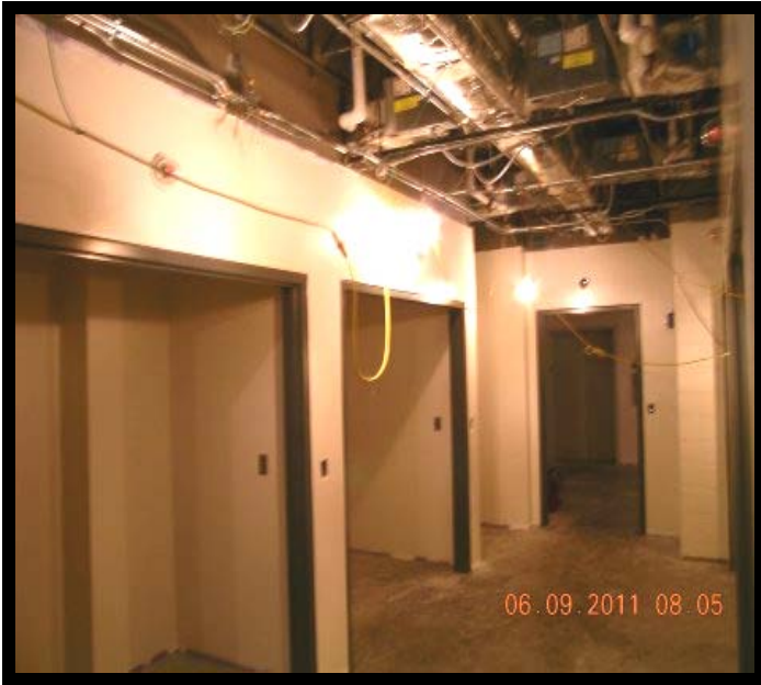
Corridors being Painted
