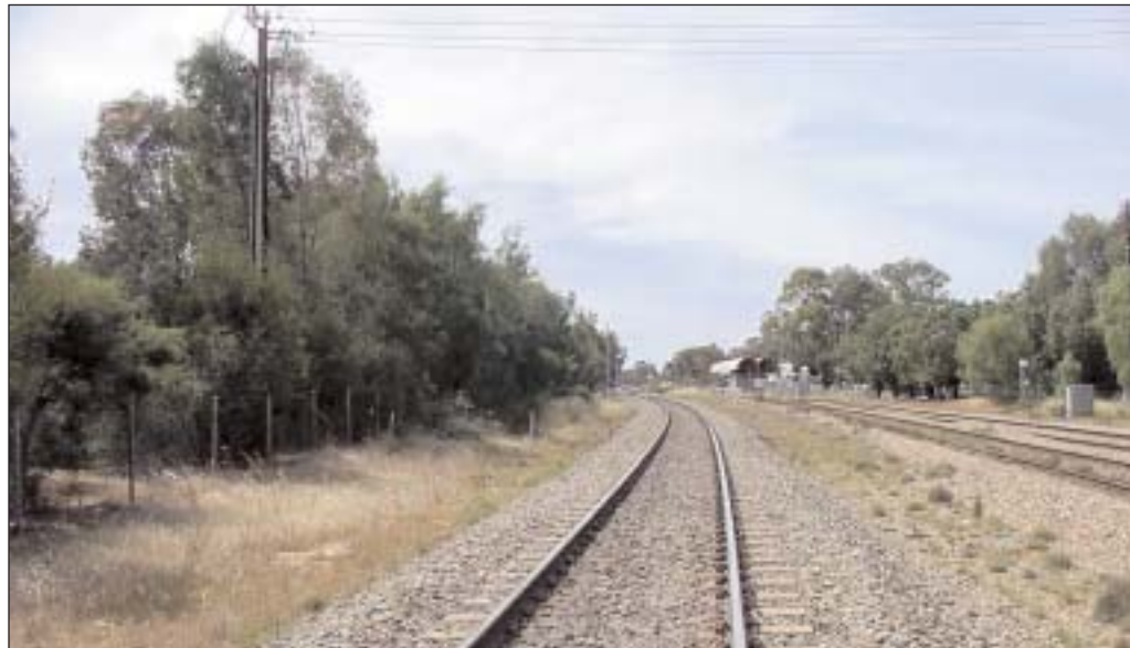
FIGURE 7: Park Terrace at about 250 m
